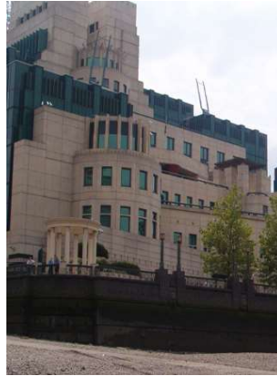
10. Which London building?
